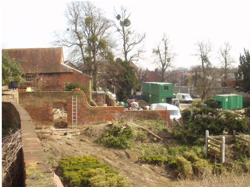
Works in progress at Caversham Court
