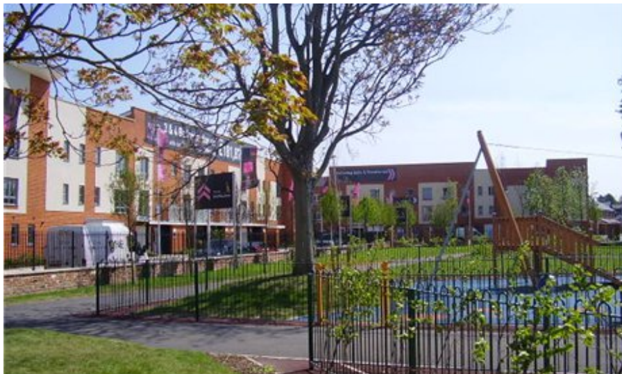
Fig. 8: New Housing development at West Village, Reading
