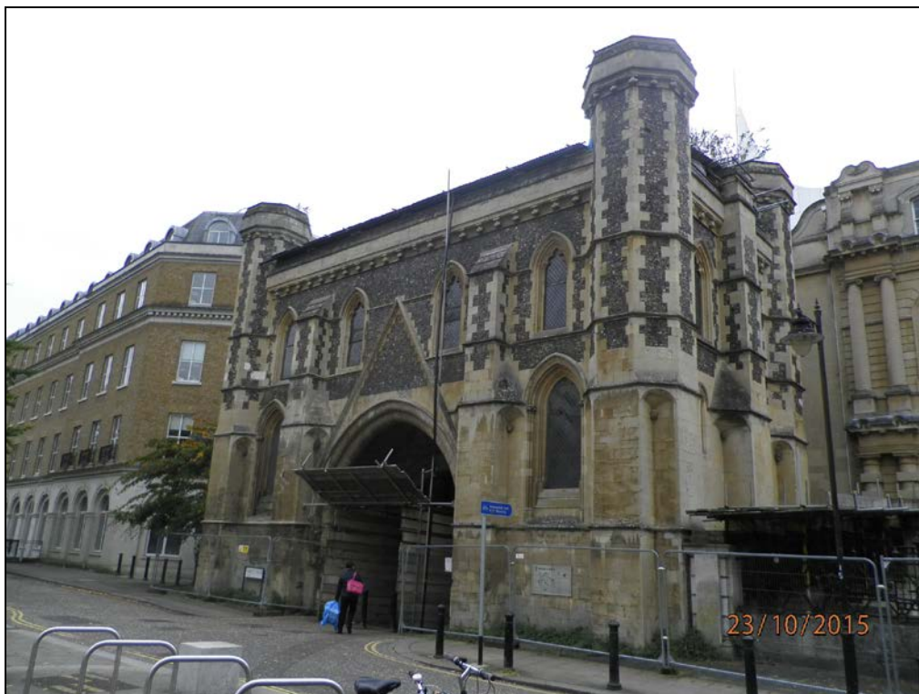
Site Photograph - north elevation to The Forbury
