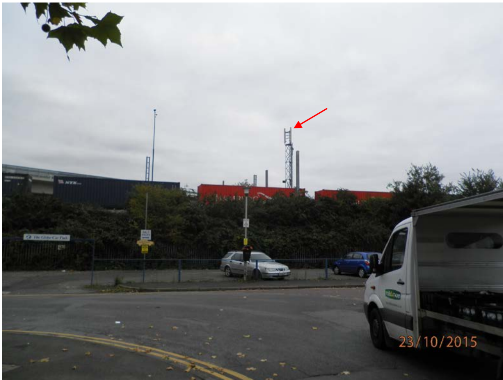
View northwards from Ashmere Terrace across Lloverock Road towards existing mast.
