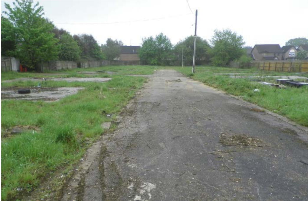
Looking south towards Orchard Grove
